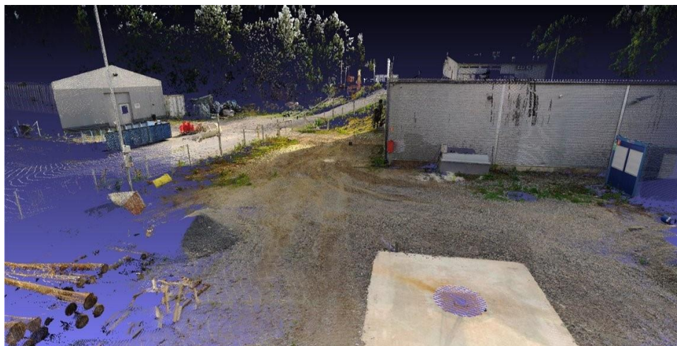
Figure 15: Processed data from the FARO Laser scanner.
